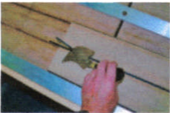
Removing top mushroom from the welded joint
